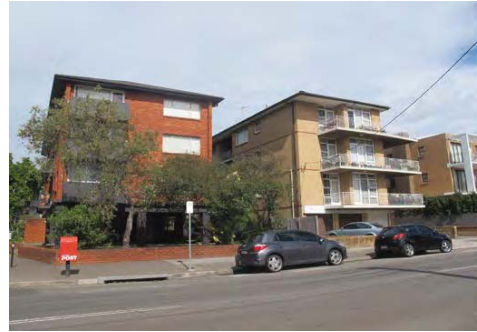
70's residential unit blocks
