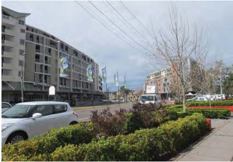
Contemporary multi-unit residential development
