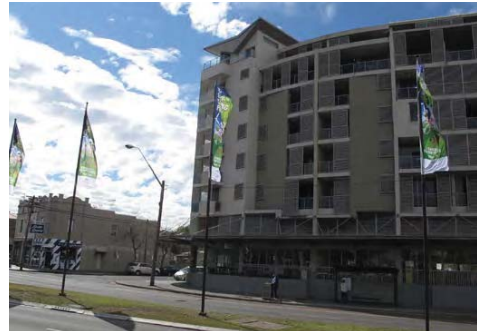
Contemporary multi-unit residential development
